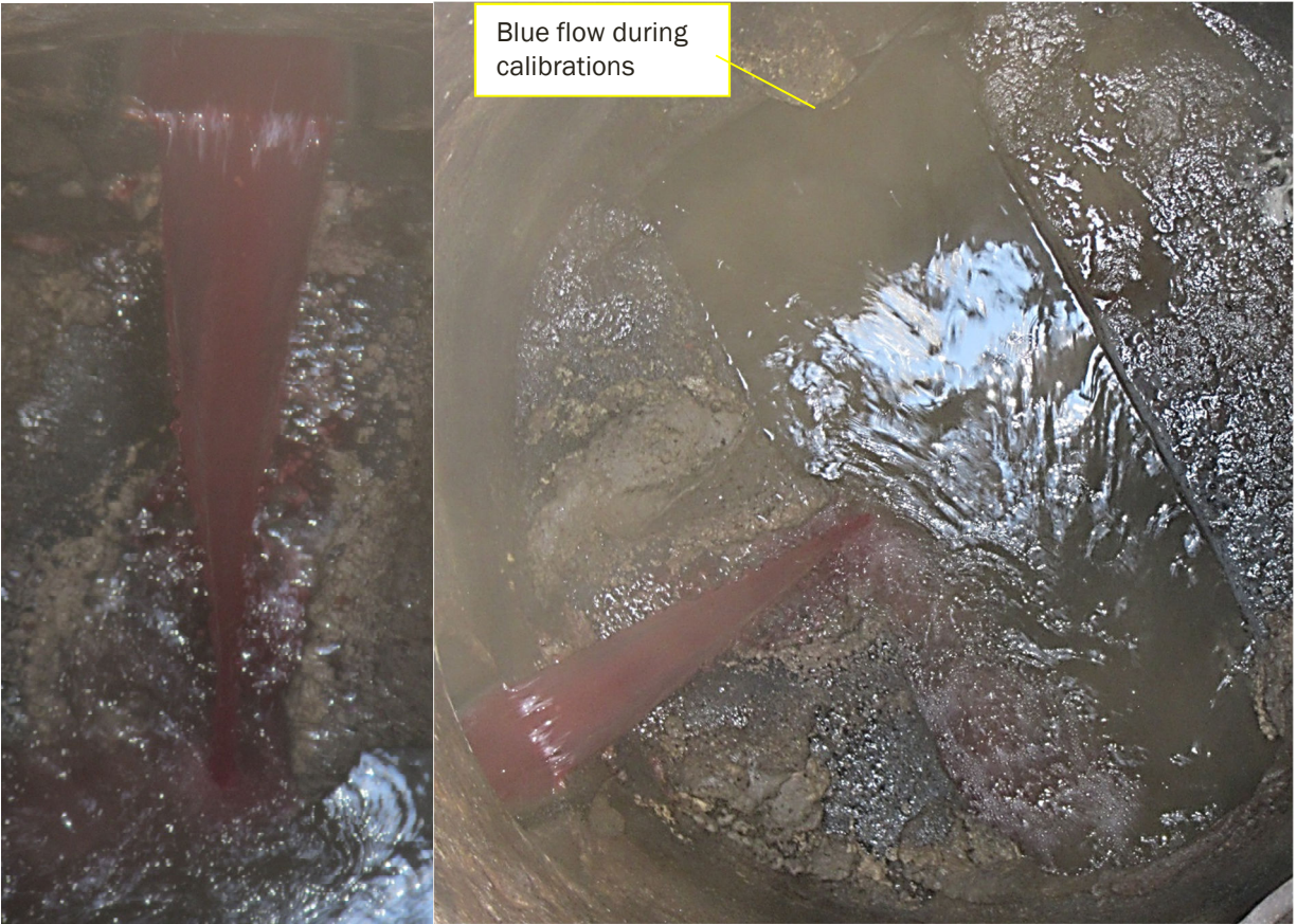
Photo 3-3. Site 7 southwest drop inlet, red flow
