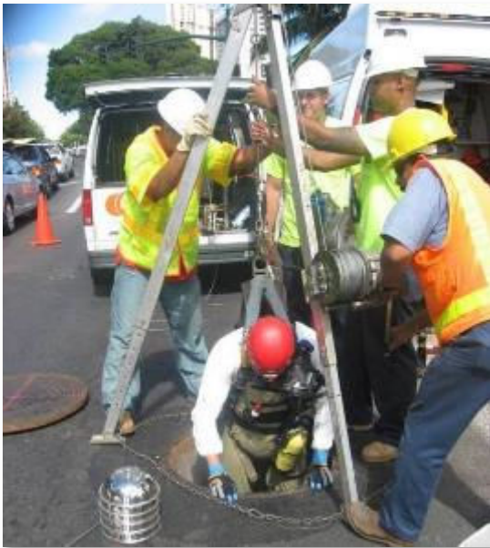
Photo 2-1. Confined Space Entry
