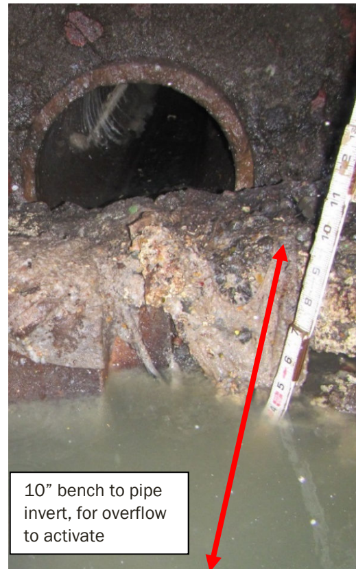
Photo 3-5. Site 9 Overflow Connection
