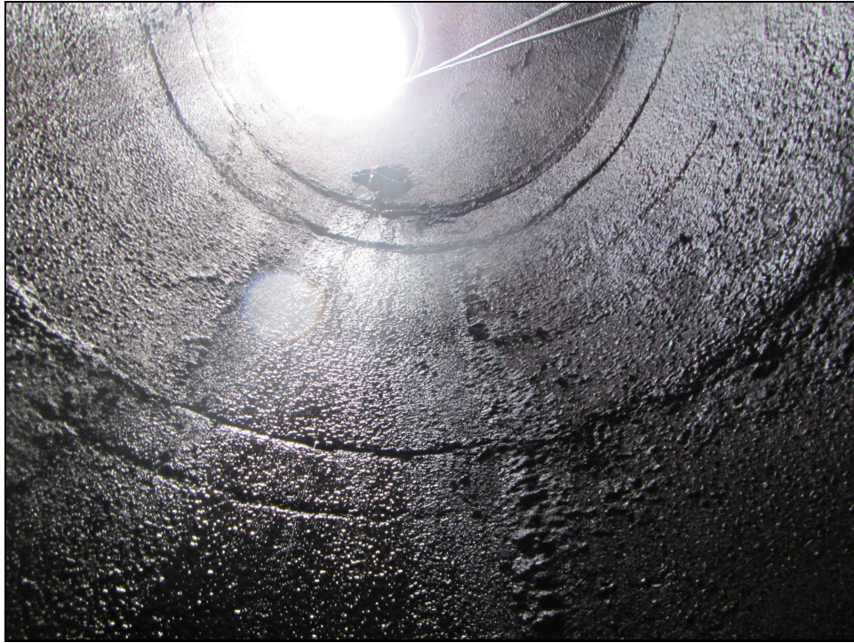
Southeast Influent Pipe
