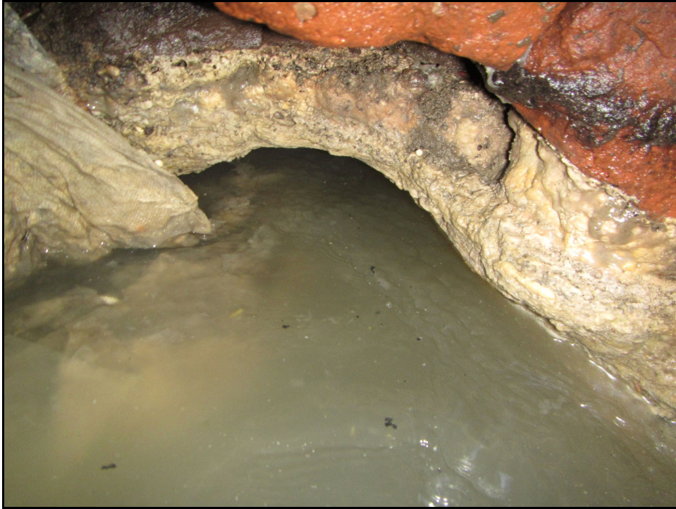
Northeast Effluent Pipe
