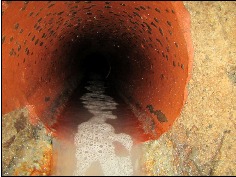
Southeast Influent Pipe
